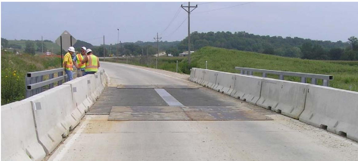
(a) Installed FRP Bridge
