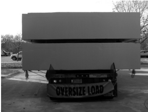
(a) FRP deck panel delivery
