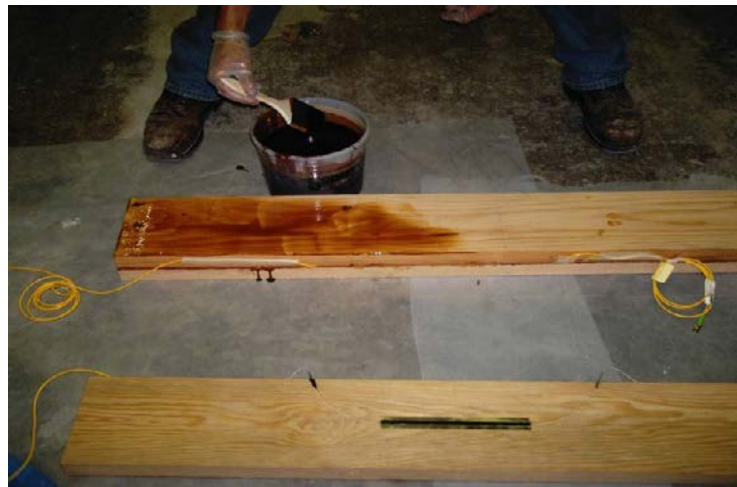
Figure 6.19. Assembly of the Glulam Specimens: Adhesive Application to Wood Laminates
