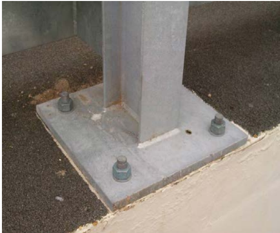
(c) Barrier rail connection
