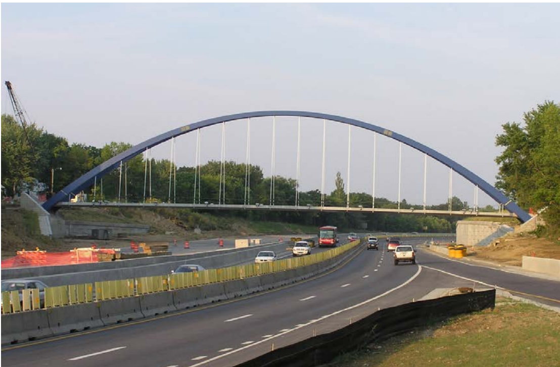
Figure 3.1. Overall View of the 40 th Street Pedestrian Bridge Over I-235 – Des Moines, IA
